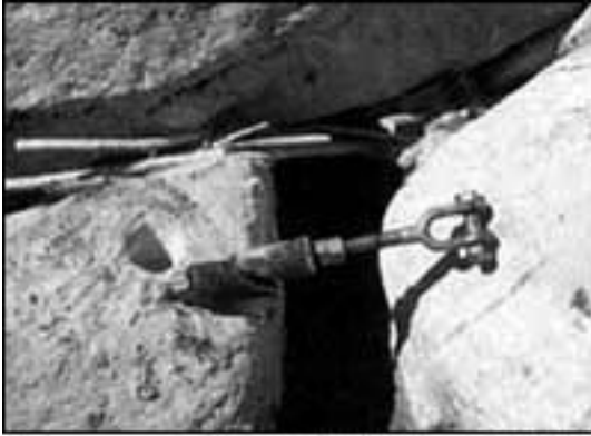
Expansion bolt next to hole
