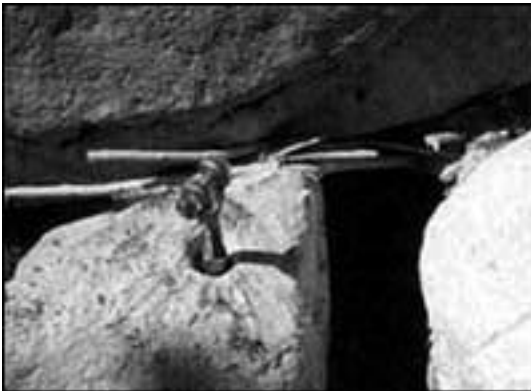
Expansion bolt placed in hole & tightened
