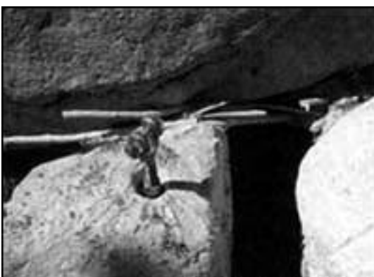
Snatch block attached to eye and ready for lift
