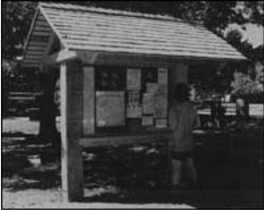
CVATMA installed the Cadillac of information boards with 10- x 10-inch oak and a hand-carved "Welcome to the A.T." at ATC's mid-Atlantic regional office in Boiling Springs, Pa. (photo by Karen Lutz)
