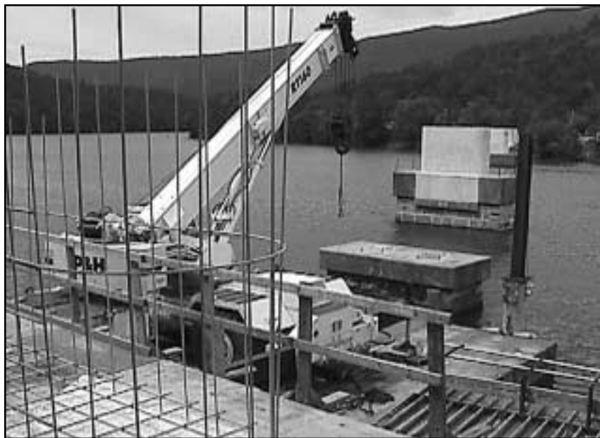
Crane and existing bridge piers.
