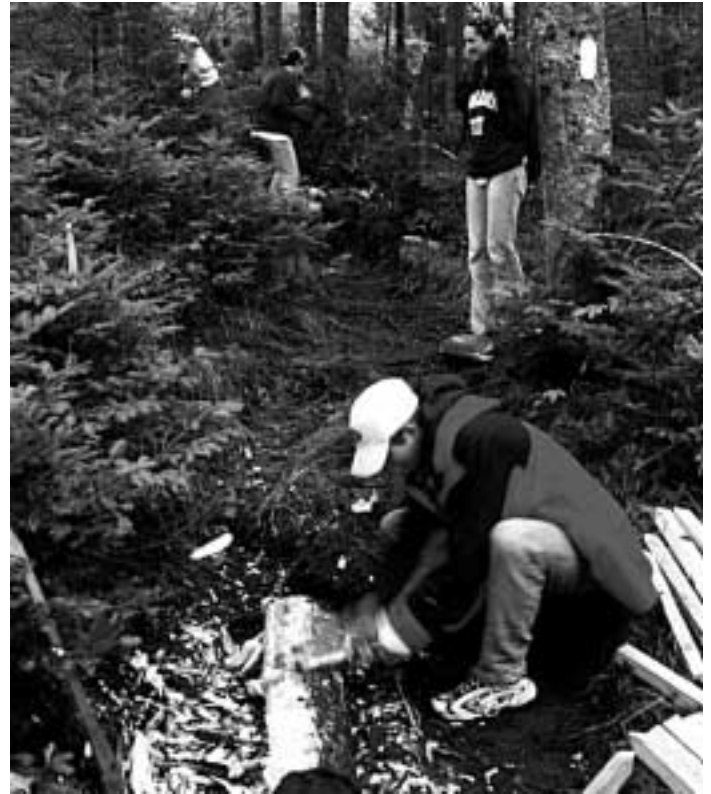
Erin McKinnon, Maranda Love, and Matt Long from ASU peeling logs and installing waterbars on Roan Mountain. (Photo by Bill Stowell)
